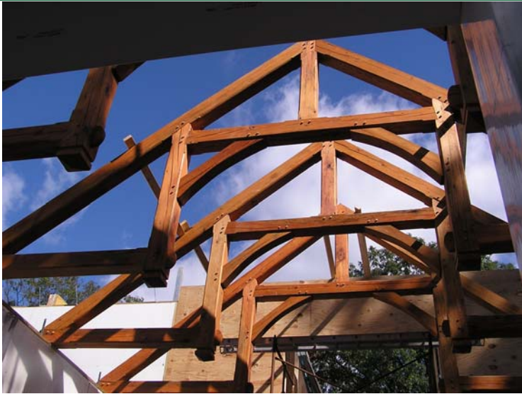
TimberFab construction of interior Timber frame trusses.
