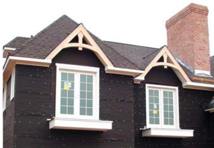
Exterior timber framing.
