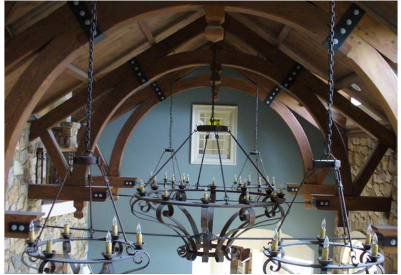
Timber Framing in Great Room of Current PAI Project.
