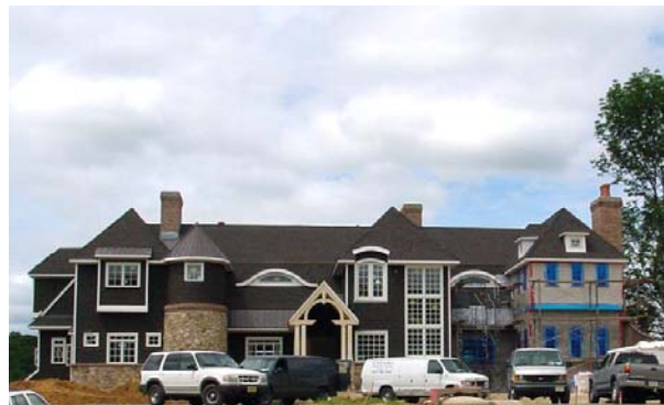
Current Progress on French Country house.
