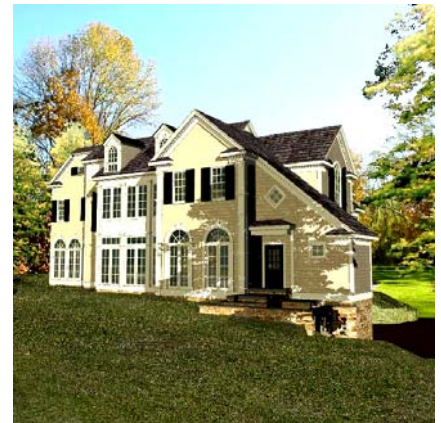
Saltbox roof line on current PAI construction.
